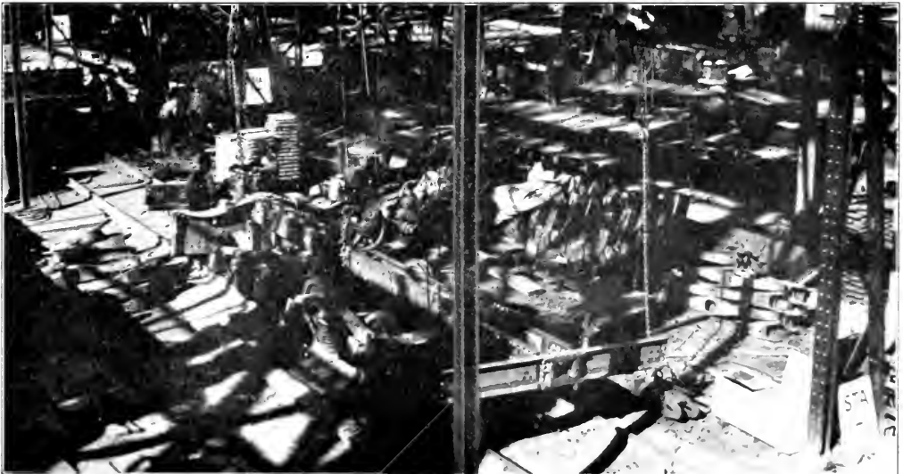
FIG. 48. ERECTING STATION No. 5 WHERE THE DRAFT GEAR IS INSTALLED
